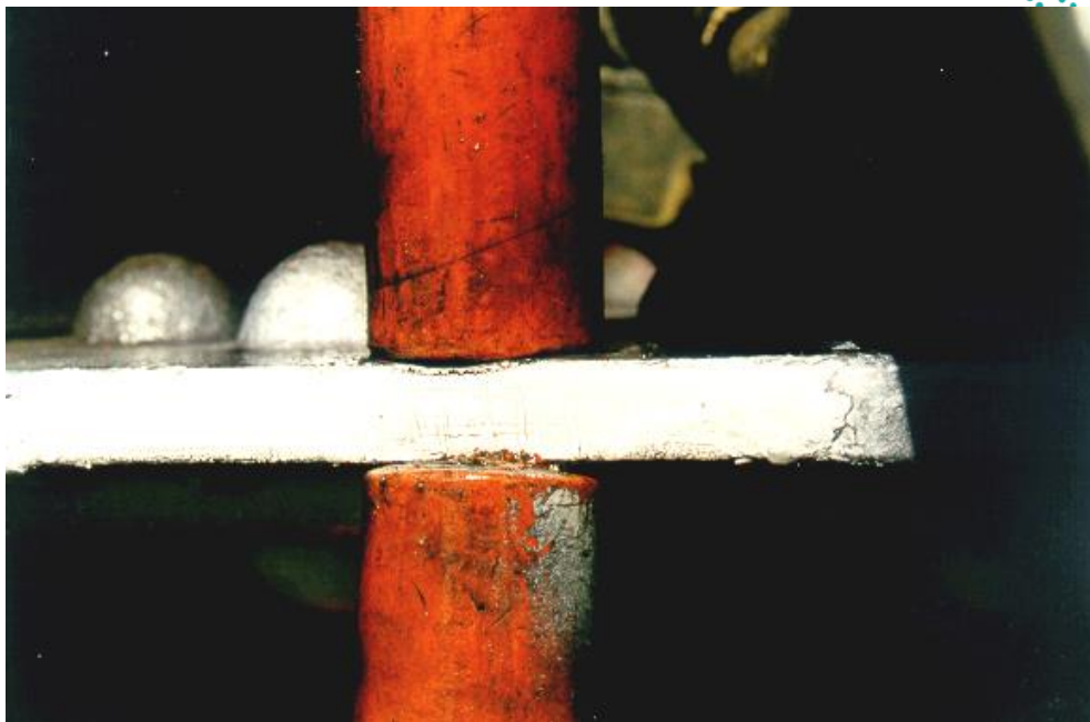
Figure 18 - Deck girder, edge filed at top flange. Laminations confirm drawing notation as wrought iron
